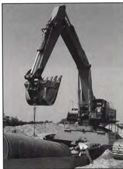
Installation Contractor, John D. Stephens, lays 60" P-303 at Lake Ivie. Project is scheduled for completion by February 1, 1995.
