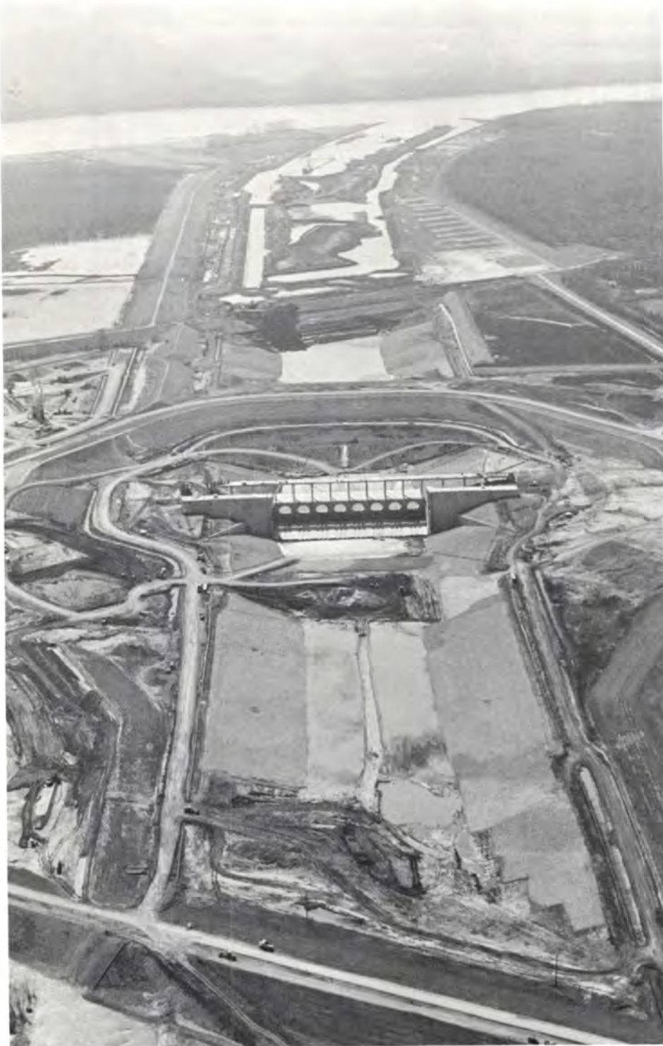
Aerial view of the Sidney A. Murray, Jr. Hydroelectric Station. The plant site is located 40 miles south of Vidalia, Louisiana, near the Old River Control Structure. After completion, Louisiana Highway 15 will be re-routed across the power channel by a bridge incorporated on top of the plant structure.
