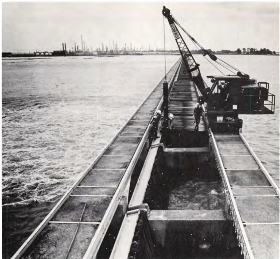
A crane atop the spillway lifts one of the 7,000 "needles" to begin opening one of Bonnet Carre's bays.
