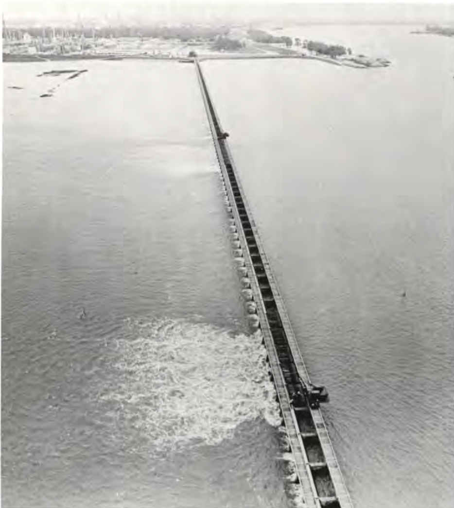
Water flows from the Mississippi River through a few of Bonnet Carre's 350 bays to Lake Pontchartrain to protect New Orleans and downstream Louisiana parishes from flooding.
