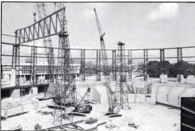
92 ton truss section for the University of Texas in Austin.
