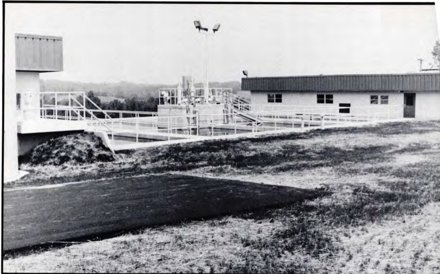
CREDITS FOR OWEN AND WHITE, INC. OUTSTANDING PROJECT—Hiwassee Utilities Water Treatment Plant
