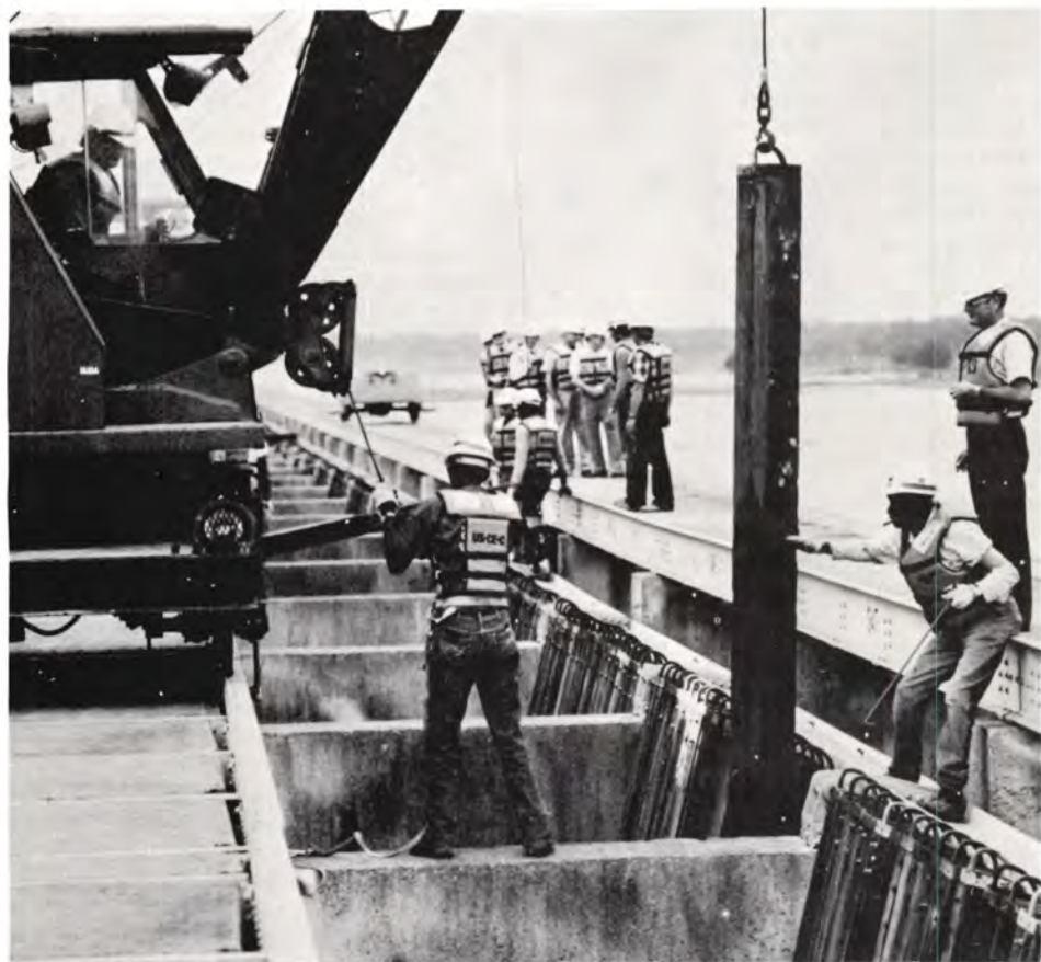
A crane atop Bonnet Carre spillway pulls an 8x11-1/2-inch timber "needle" from a bay.
