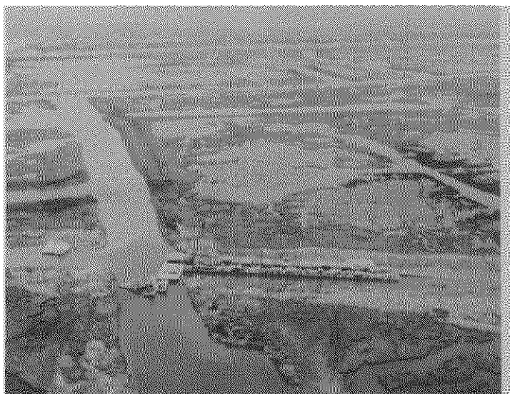
Crude pipeline construction (48" diameter).
