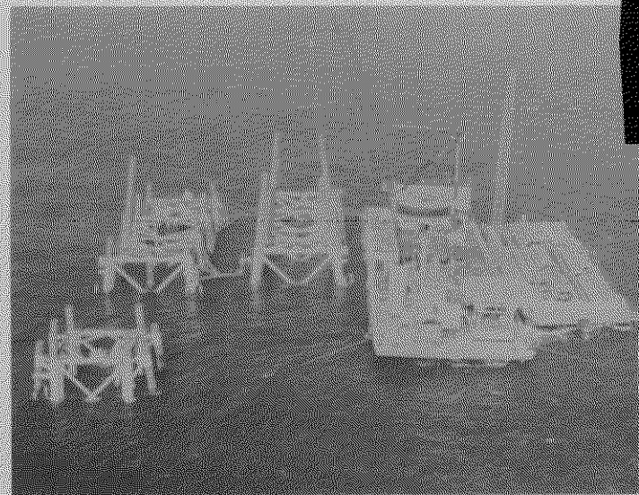
Jackets installed for offshore platform.
