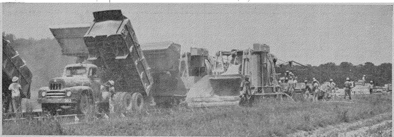
Split-second coordination plus high-speed equipment keeps three mixers working abreast, setting new paving pace for Louisiana highway construction.
