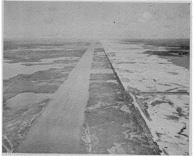
VAST AREAS of typical Louisiana marshland along the route of the Mississippi River-Gulf Outlet have been changed into high areas that will be ideally suited to industrialization. One such area where dredged material was placed between retaining dikes can be seen in this view along the right descending bank of the channel.
