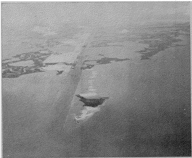
GUARDING the new $95 million Mississippi River-Gulf Outlet's entrance into Breton Sound are two 3 mile long stone dikes. More than 20 miles of the channel are visible in this photo. The light areas on the left of the channel are spoil disposal areas, now raised to an elevation of several feet above sea level.
