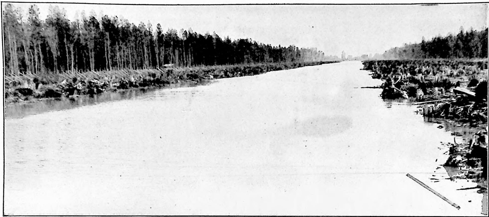
FIG. 3 VIEW OF CANAL AFTER EXCAVATION
