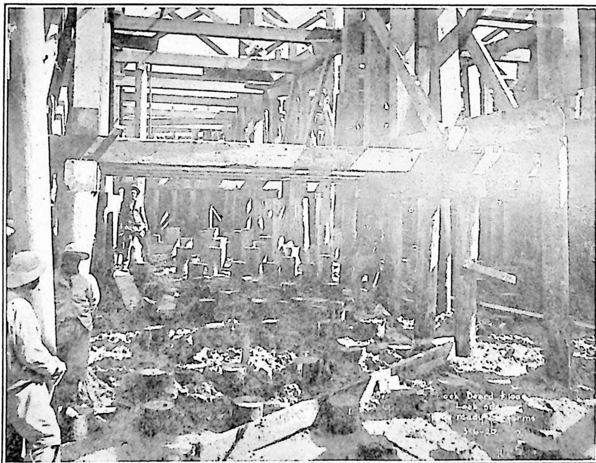
FIG. 7. CROSS BRACING AND FINISHED SECTION OF LOCK EXCAVATION
