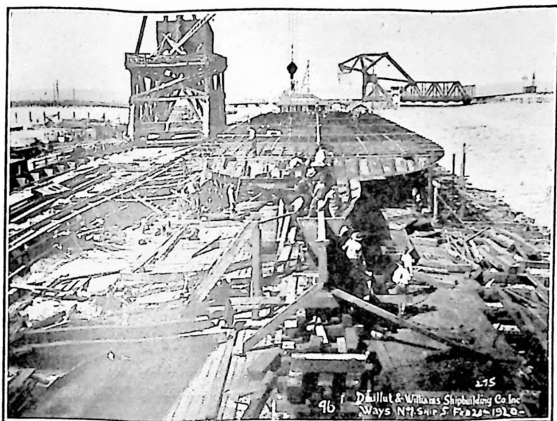
HULL NO. 5. THREE WEEKS AFTER THE LAUNCHING OF THE "NEW ORLEANS" FROM THESE WAYS
