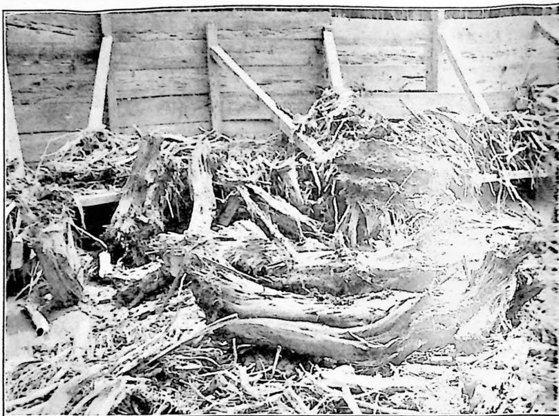
FIG. 5 STUMPS AND ROOTS HANDLED AND ACTUALLY PUMPED BY THE DREDGE Texas
