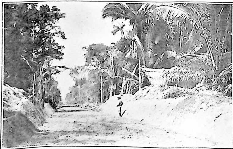
COMPLETED SUB-GRADE FOR RAILROAD. ADJOINING LANDS TO BE CLEARED AND PLANTED IN BANANAS.
