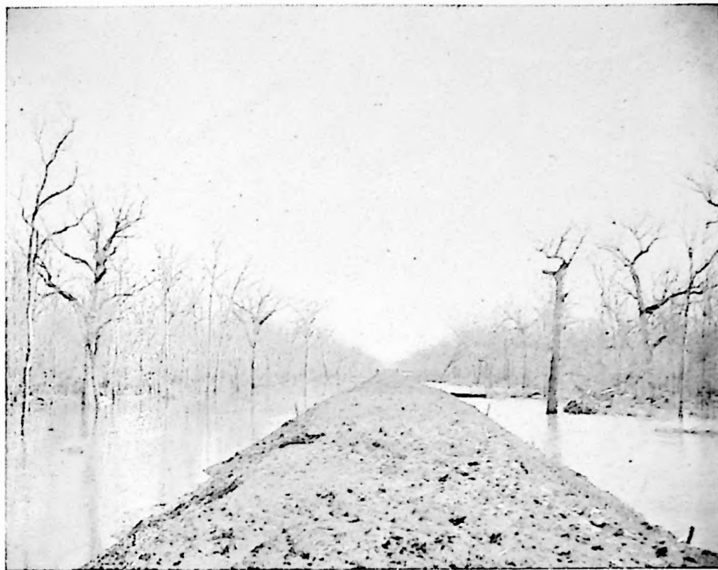
EARTH ROAD IN PROCESS OF CONSTRUCTION THROUGH A SWAMP CALDWELL, PARISH
