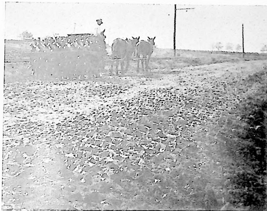
ASPHALT-GRAVEL ROAD JUST AFTER BEING GRADED NEW IBERIA—JEANERETTE
