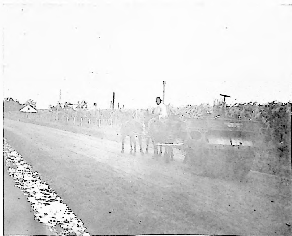
ASPHALT-GRAVEL ROAD. FIRST LIGHT ROLLING. NEW IBERIA—JEANERETTE.
