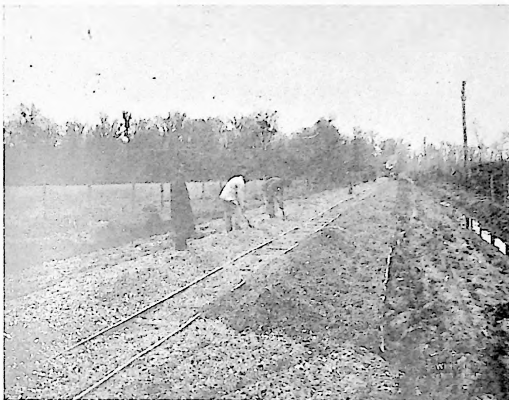
GRAVEL ROAD IN PROCESS OF CONSTRUCTION BATON ROUGE—HOPE VILLA
