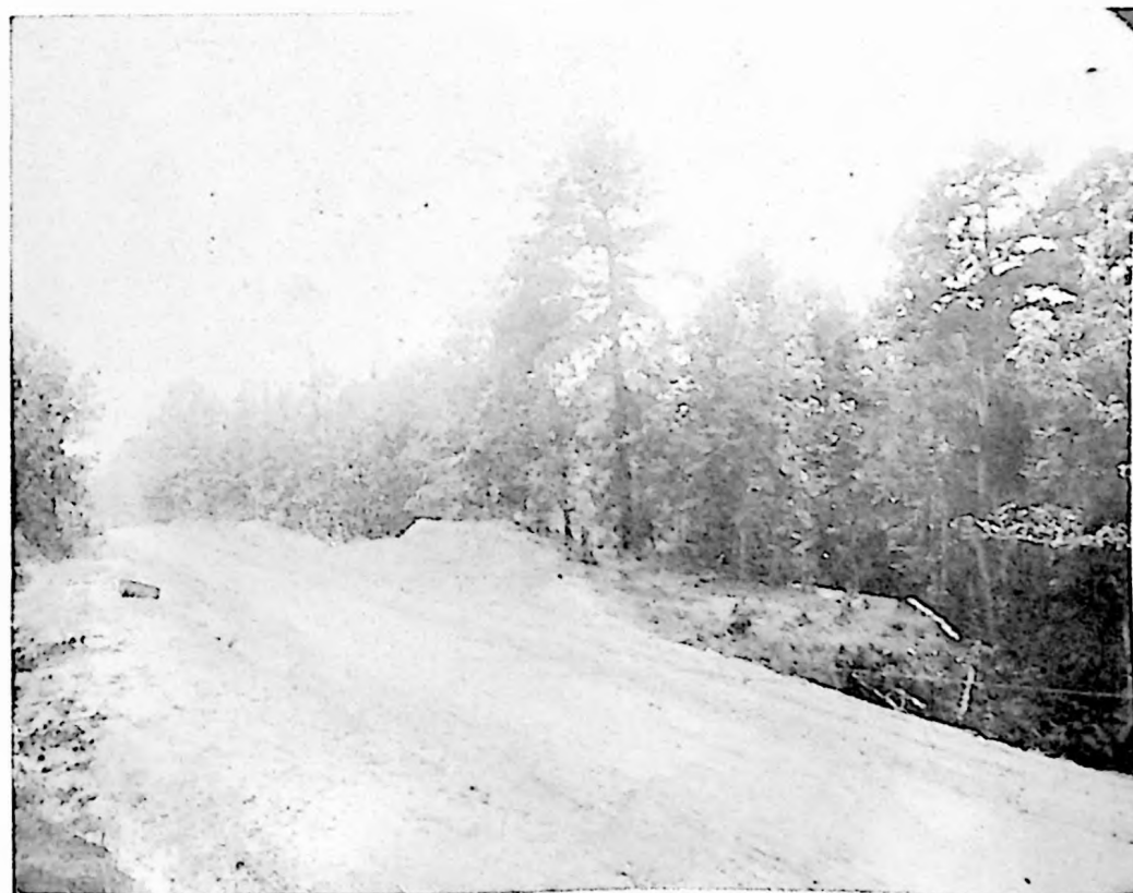
THE SAME ROAD COMPLETED
