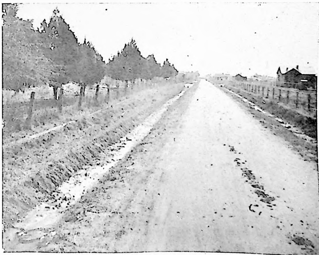
THE SAME ROAD COMPLETED
